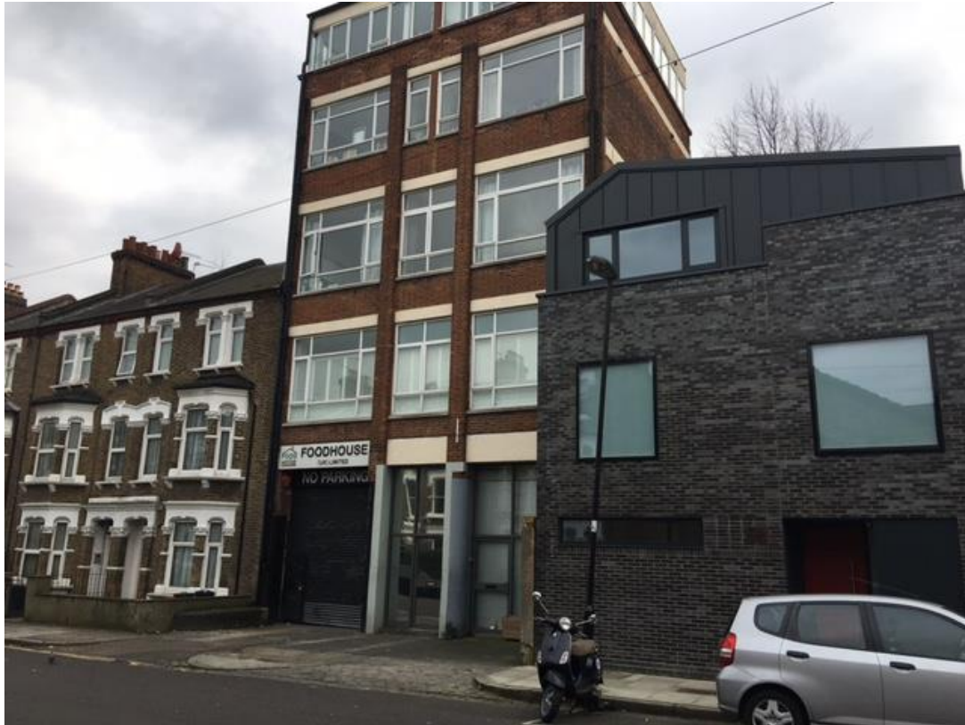
2a Fairbridge Road (with the ground floor entrance to 724 Holloway Road behind the shutters)
