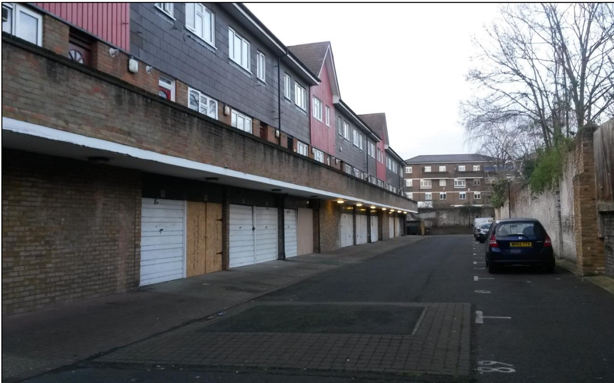
Fig. 6: Garages underneath 76-98 Surr Street (“Site 2e”)
