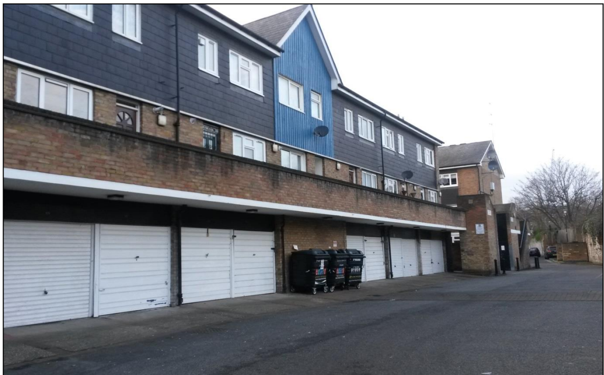
Fig. 5: Garages beneath 43-52 Surr Street (“Site 2c”)
